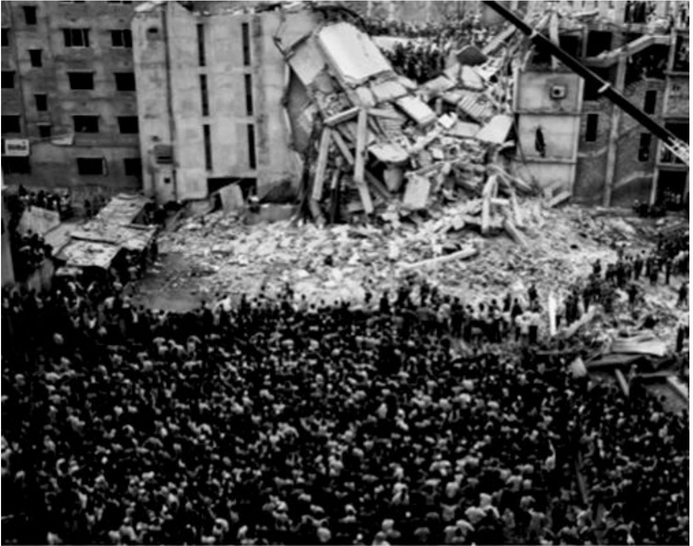
The Rana Plaza factory building shortly after it collapsed on April 24, 2013. More than 1,100 people were killed. (Photo by Ayon Rehal)
